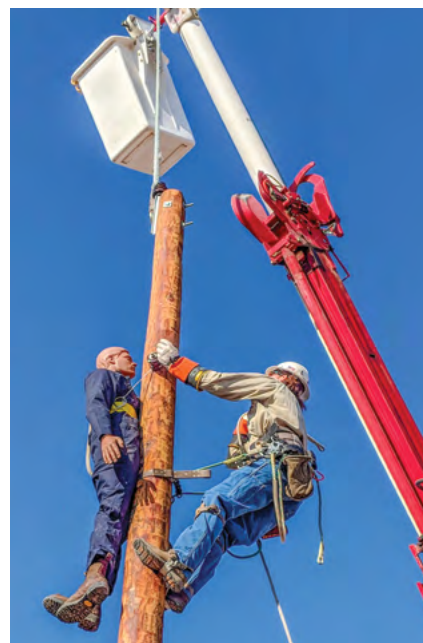
Parker Flemming, Garden City, climbs a pole to assist "Rescue Randy" during pole top rescue training.
